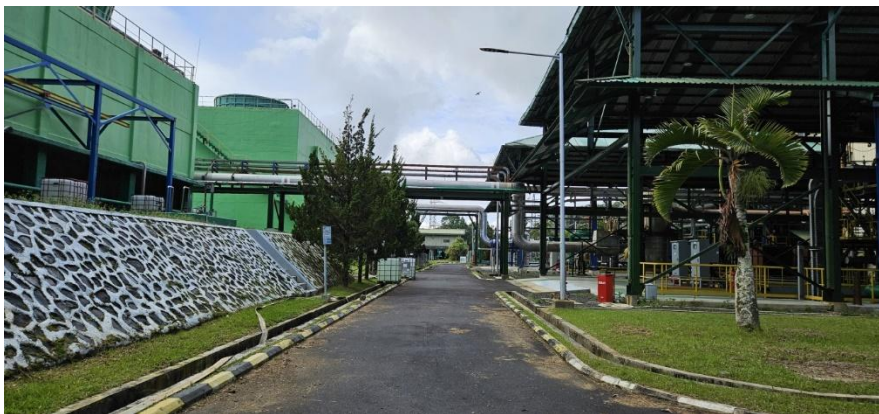
Gambar 7. Area cooling tower (Dokumentasi tim, 2025)
